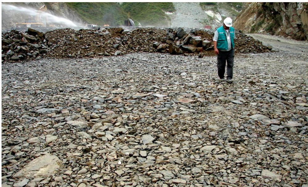
Compacted rockfill (construction of Mazar dam in Ecuador)
