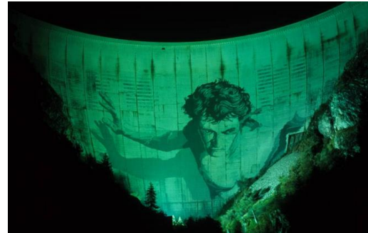
© Photo EDF A. Pellorce
