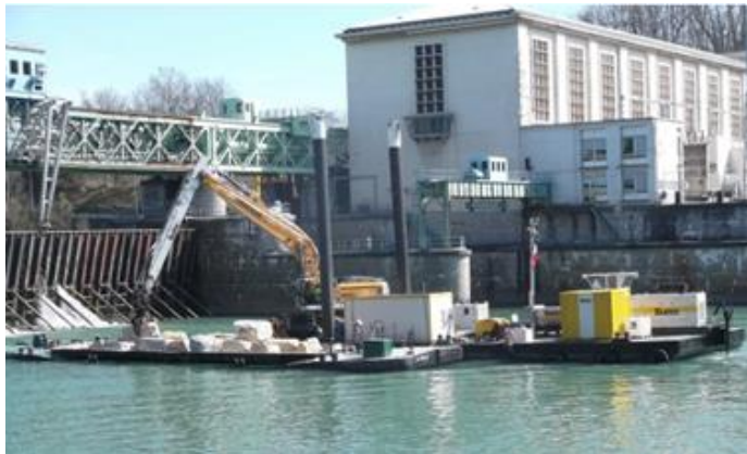
© Photo CNR Rockfill Protection works 2014
