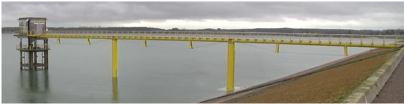
© Photo EPTB SGL Intake tower after renovation 2021
