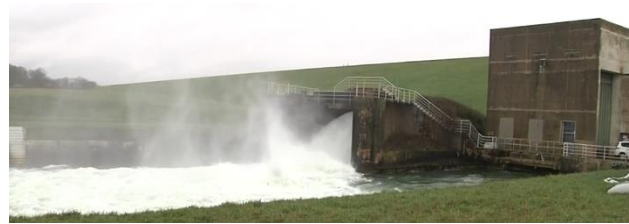
© Photo EPTB SGL Morge gallery exit in operation
