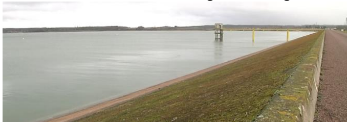
© Photo EPTB SGL Barrage de la Morge
