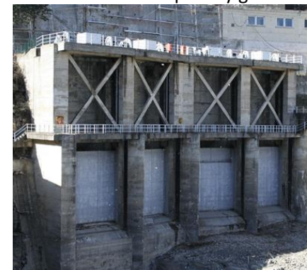
© Photo EDF Surface spillway on dam crest
