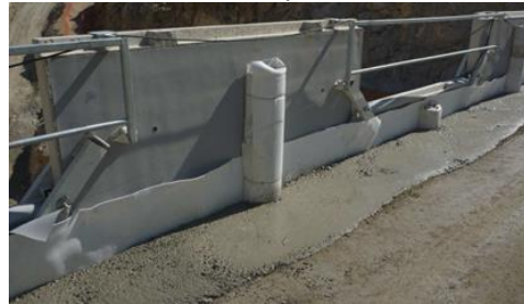
© Photo EDF upstream face
