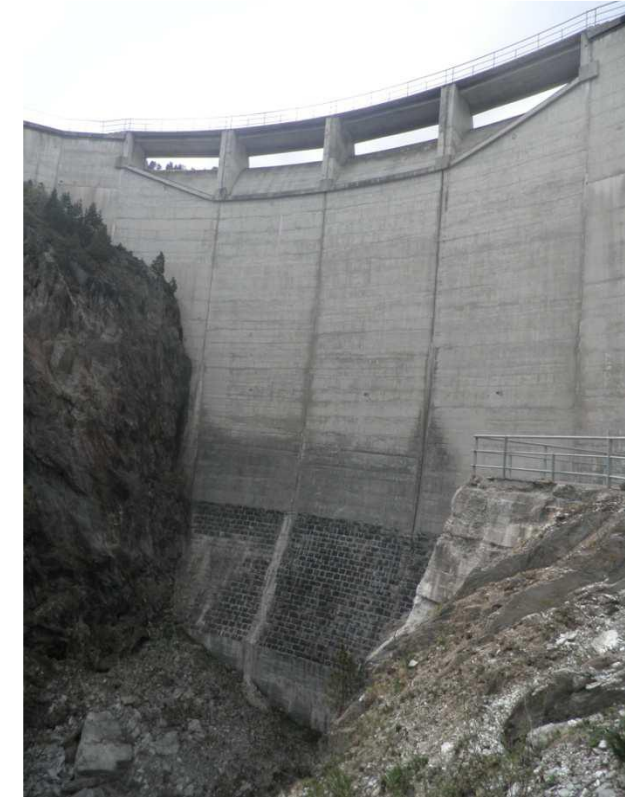
© Photo EDF Arch dam
