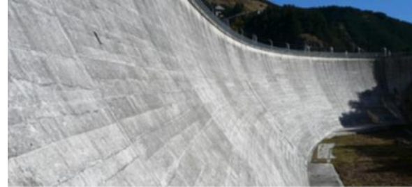
© Photo EDF Gravity dam
