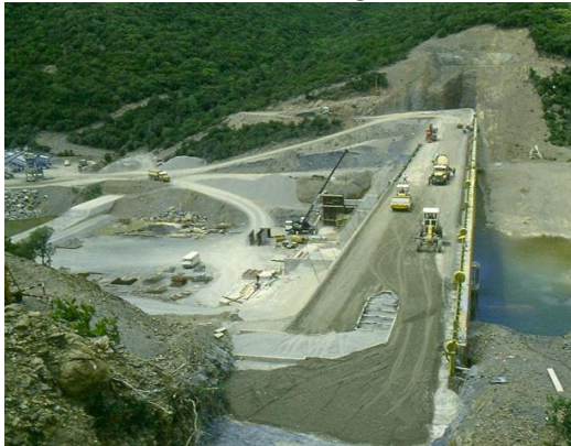
© Photo BRL Ingénierie Open sluiceway in operation
