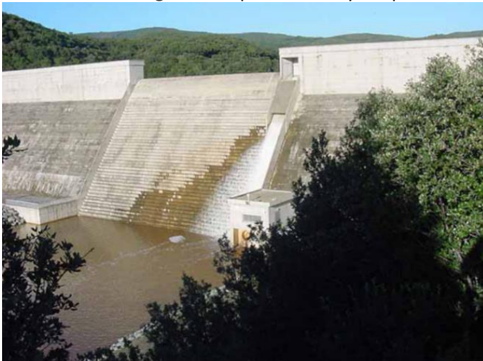
© Photo BRL Ingénierie Open sluiceway in operation
