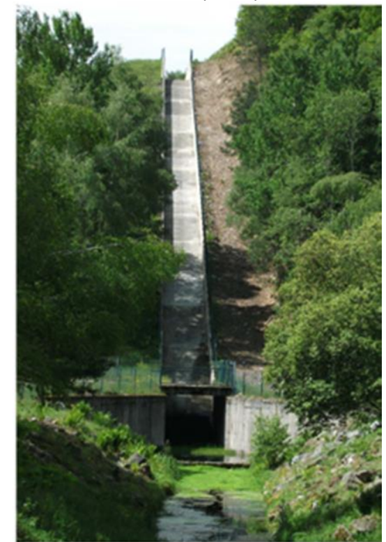
© Photo EDF Spillway chute
