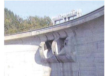
© Photo EDF downstream view
