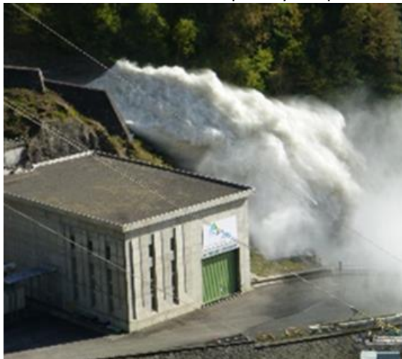
© Photo SHEM Left bank spillway in operation
