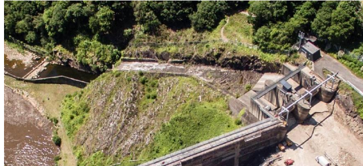
© Photo EDF spillway general view
