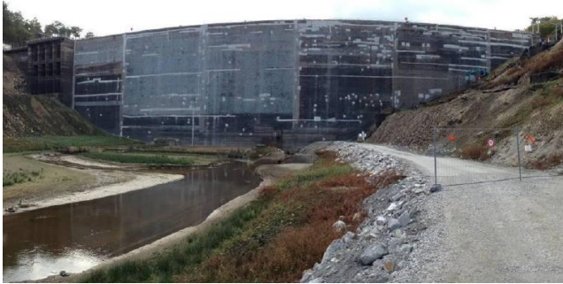
© Photo EDF dam upstream view
