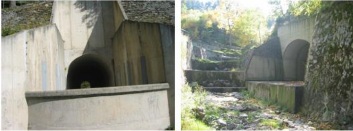
© Photo EDF F. Delorme main spillway (1)
