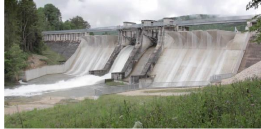
© Photo EDF P. Valley rehabilitated dam in operation
