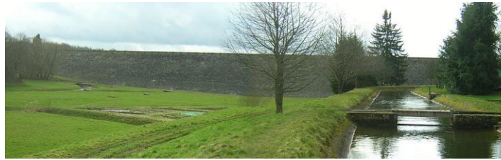
© Photo CC BY-SA 3.0 downstream view
