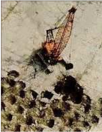
Figure 8-2 – Compactage dynamique
