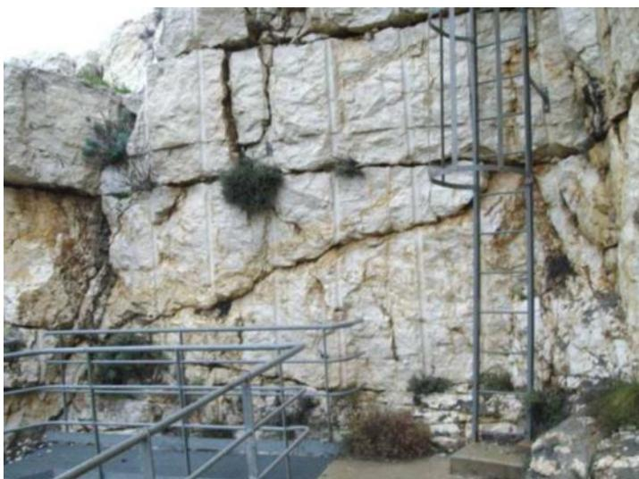
Figure 2.9 –Geological inspection of unstable blocks on one of the dam sides
