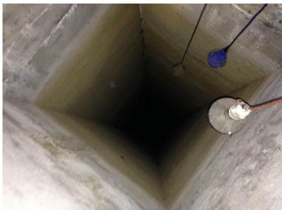
Figure 2.3 – Checking the position of water level alarm switches in a shaft
