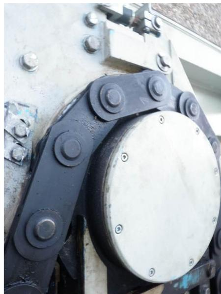
Figure 2.6 – Inspection of the state of the Galle chain of a spillway gate
