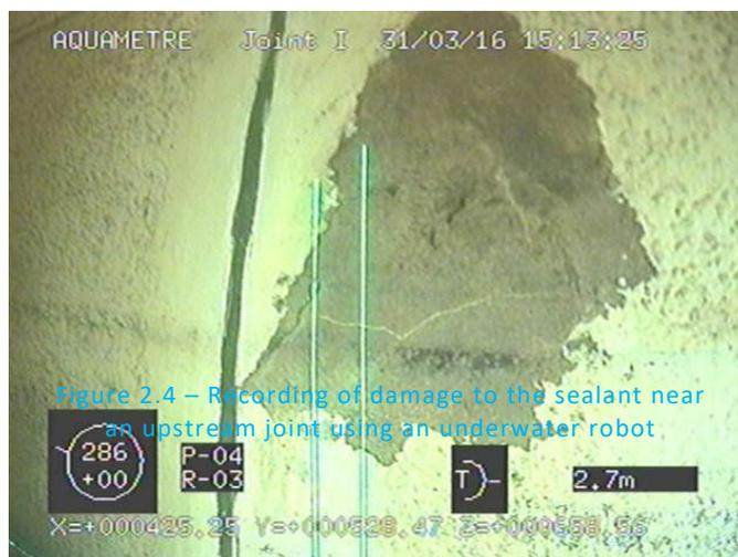
Figure 2.4 – Recording of damage to the sealant near an upstream joint using an underwater robot
