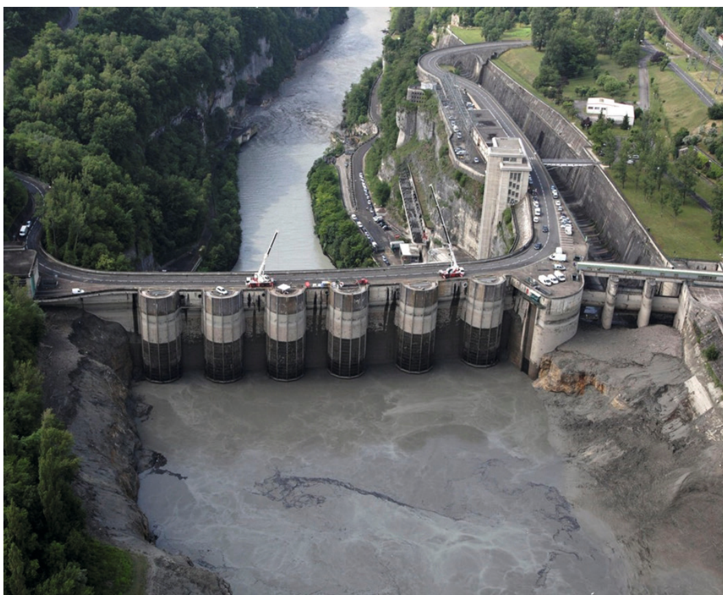
Figure 4.1 – Controlled lowering of the water level in the Génissiat reservoir during Swiss flushing operations in the Upper Rhône in 2012 / © CNR – Camille Bezzina
