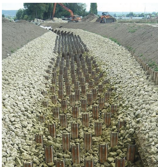
Figure 8.17 – Photograph of macro-roughness out of water and in water / © BRLi
