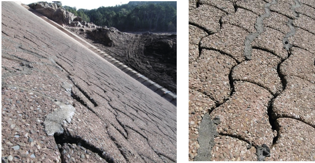
Figure 7.8 – Bulging (left) – Exposed aggregates and mortar leaching (right) /
