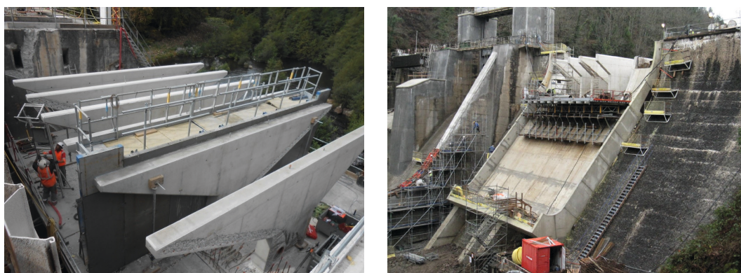
Figure 3.8 – (a) Record dam on the river Agout (2015) – Four radial gates were replaced with four piano key weirs (PKW) following the installation of a temporary protective cofferdam enabling the dam to be kept in operation, (b) PKW being fitted on Étroit dam (2009) / © EDF – F. Laugier
