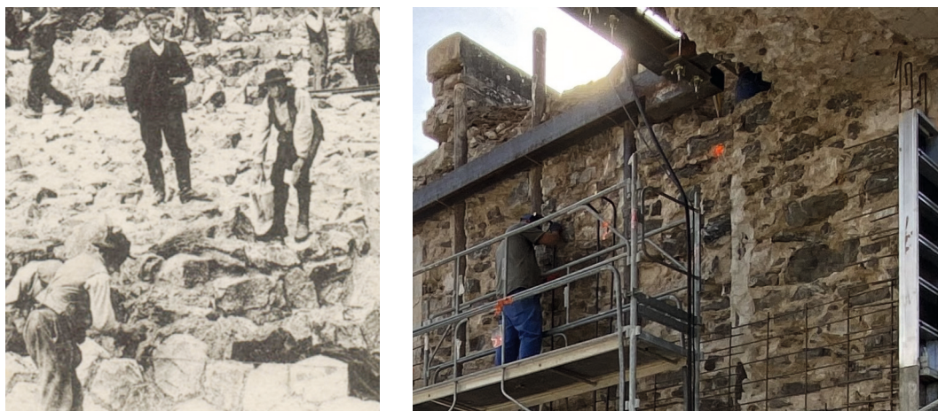
Figure 5.5 – Heterogeneity of block size and mortar filling, Rochebut & Chazilly /
