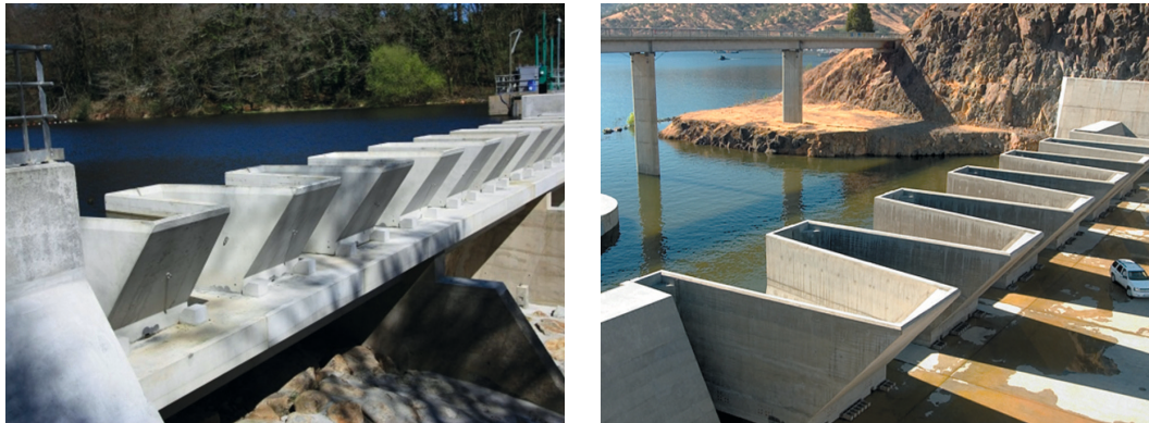
Figure 3.9 – Concrete fusegates on Tréauray dam in France (2014) and Terminus dam in the USA (2004) / © Hydroplus
