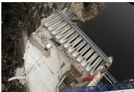
a) PKW of Malarce dam Completed PKW
