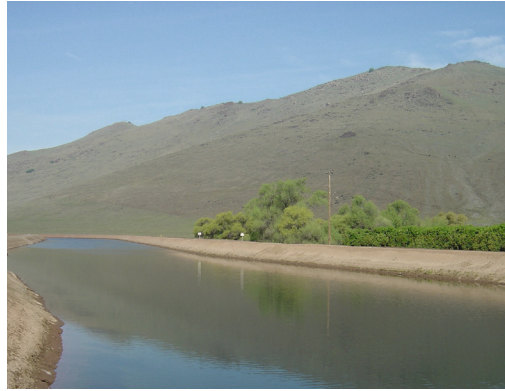
Figure 7.11 – Friant Kern Canal (USA, 2012) – Section of embankment rehabilitated in 1973 by lime treatment of swollen soils, without a concrete protection slab / @ Lhoist
