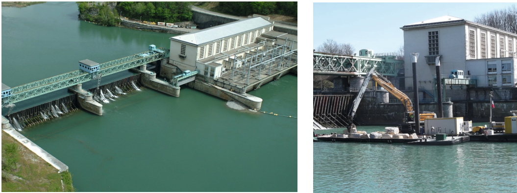
Figure 8.8 – Seyssel barrage – Aerial view and riprap works / © CNR
