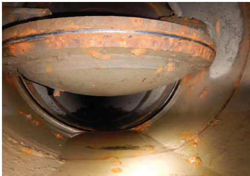
Figure 12.4 – Examination of the condition of a butterfly valve lens in a bottom outlet / © EDF
