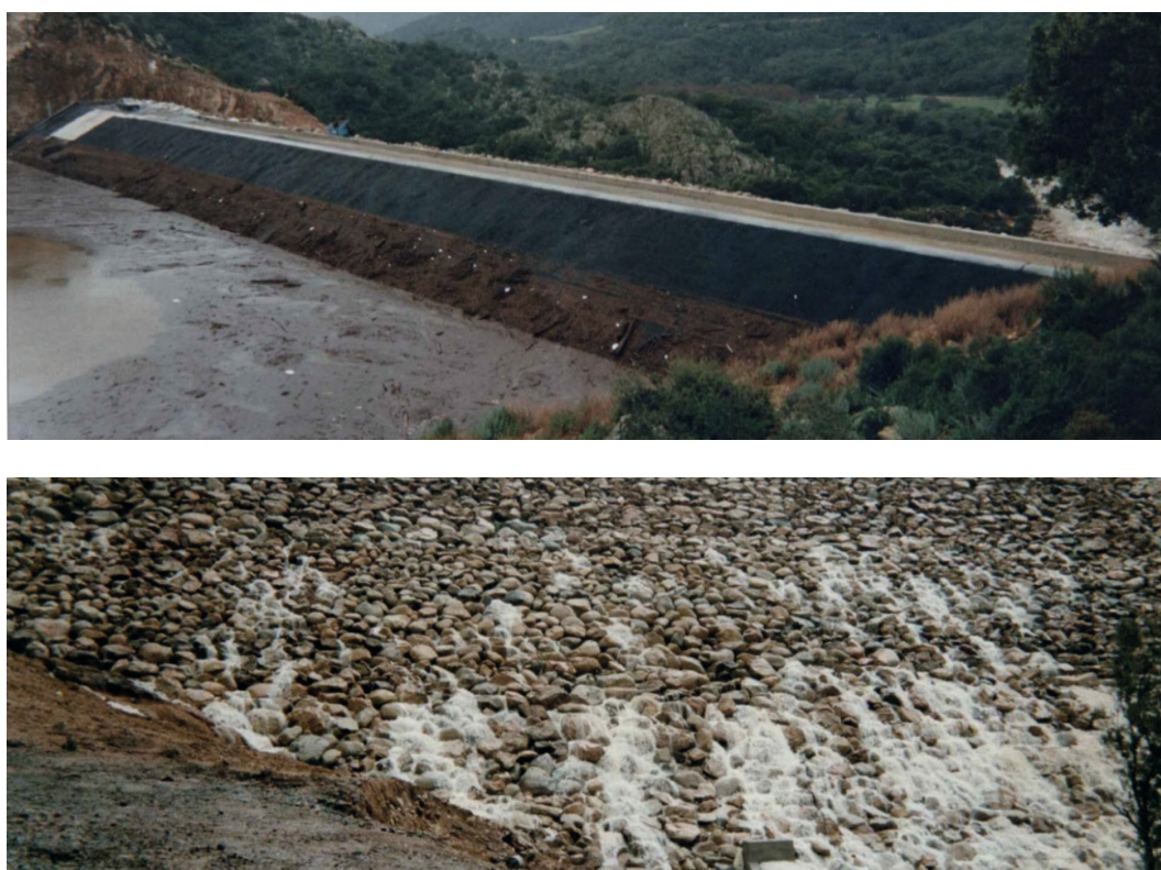
Figure 7.9 – Ortolo dam: extreme flood during construction. Upstream face (top) and downstream (bottom) / @ A. Sanguinetti
