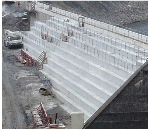
Figure 5.11 – Rassisse dam, stabilization by concrete backfill (left: before; right: after) / © ISL – Anthony Dols
