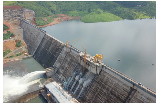
Souapiti (Guinea) – 2020 H = 110 \text{ m} - V = 4 \text{ hm}^3 © TRACTEBEL
