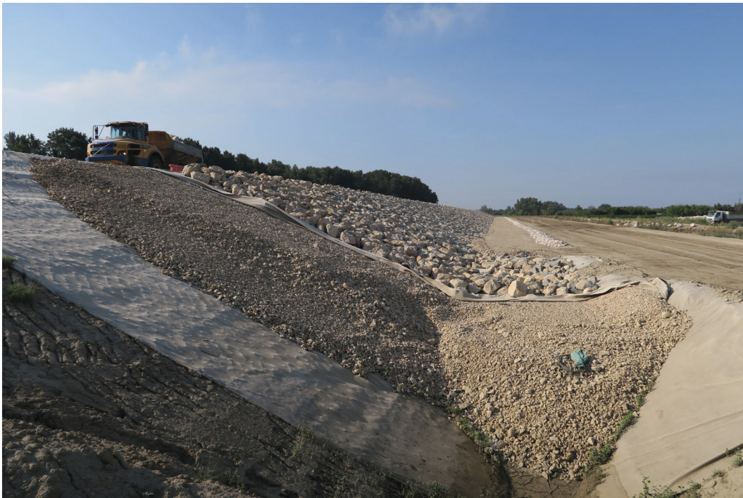
Figure 9.2 – Construction of an overflow resistant levee with all the components needed for its safety and durability (watertightness, filtration, drainage, spilling) /
