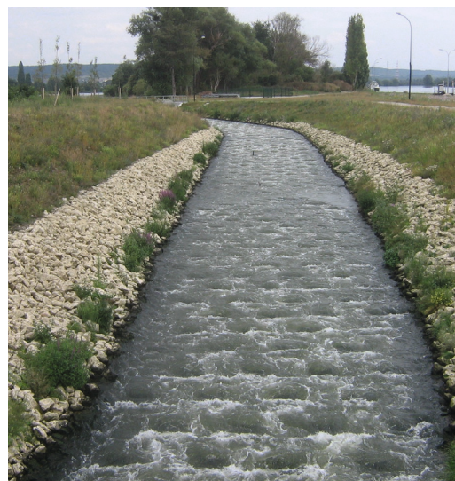
Figure 8.17 – Photograph of macro-roughness out of water and in water / © BRLi
