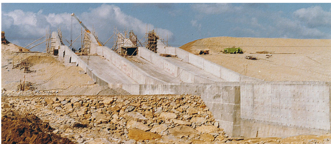
Figure 7.6 – Lebna dam: downstream face and its spillway / @ Coyne et Bellier
