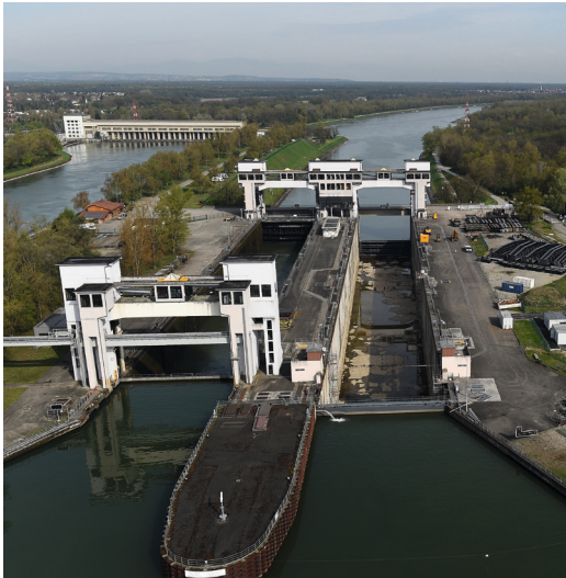
Figure 8.4 – Replacement of gates downstream of the lock chambers /
