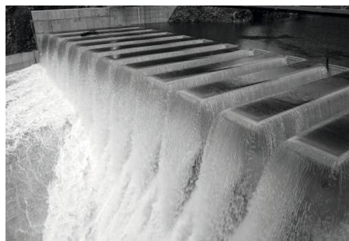
(b) During overtopping
