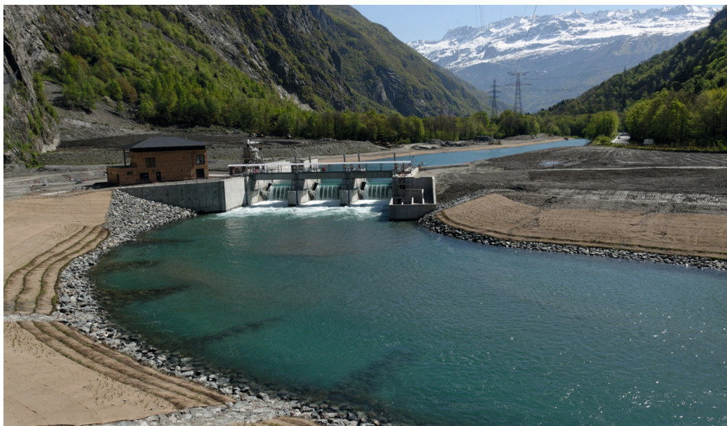
Figure 8.18 – The Livet barrage and water intake / © EDF-Christophe Huret
