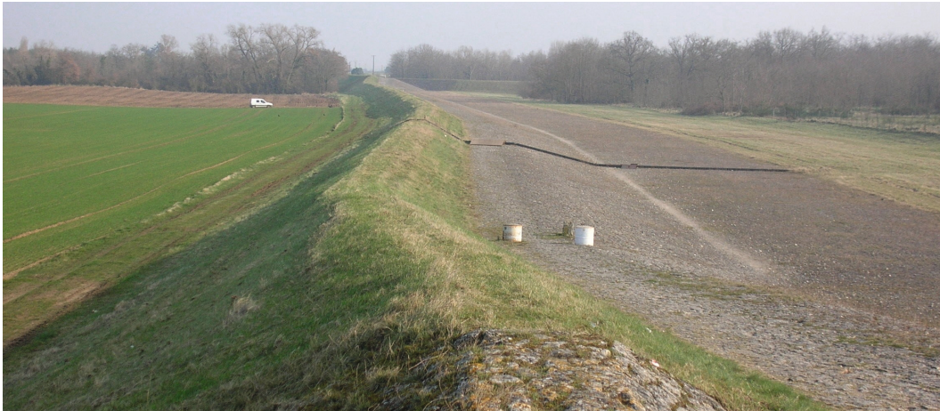
Figure 9.4 – Spillway of Jargeau (Val d'Orléans 45): from left to right unprotected area, fuse, non-erodible downstream slope, dissipation zone and protected valley /
