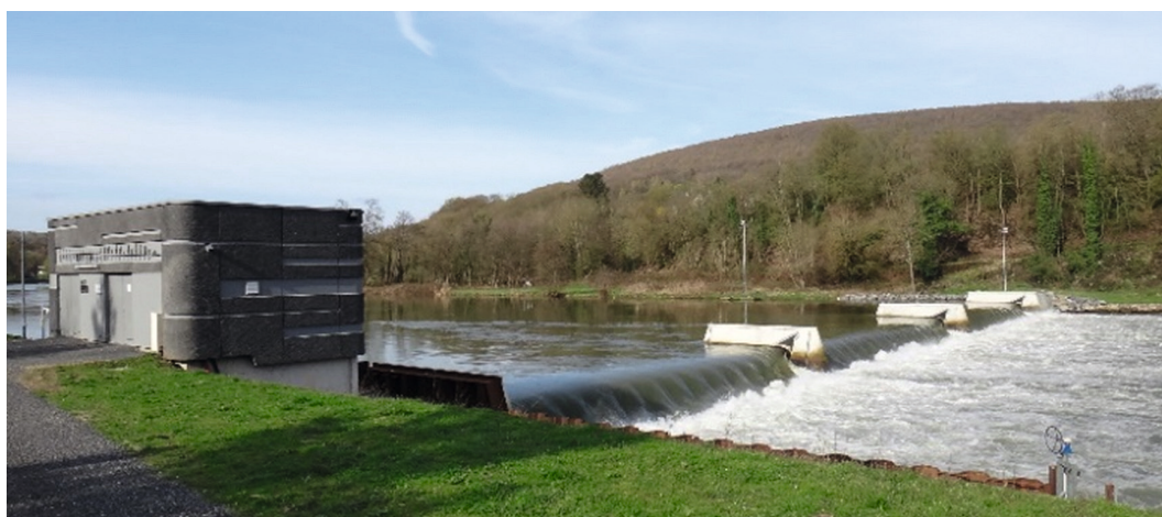
Figure 8.14 – Fépin barrage brought into service on February 2017 / © BRLi
