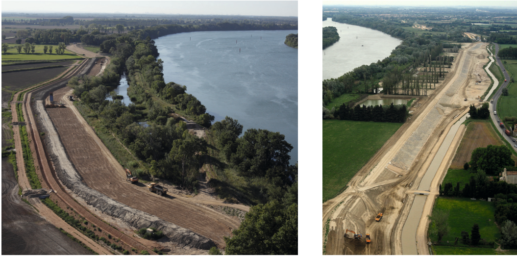
Figure 9.1 – Strategic setback south of Arles (left) and construction of an overflow resistant levee (right) / © Symadrem
