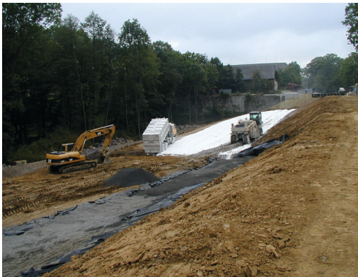
Figure 7.12 – Hvezda dike (Czech Republic, 2003) – Following floods, treatment of wet sediment with lime for dike reconstruction / @ Lhoist
