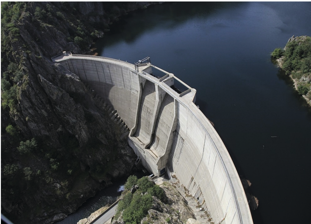
Figure 6.4 – Puylaurent, the last arch dam built in France in 1996 / © EDF – Claude Fougérol
