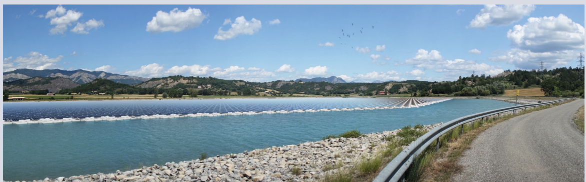
Figure 4.10 – Lazer hydropower reservoir / © EDF
