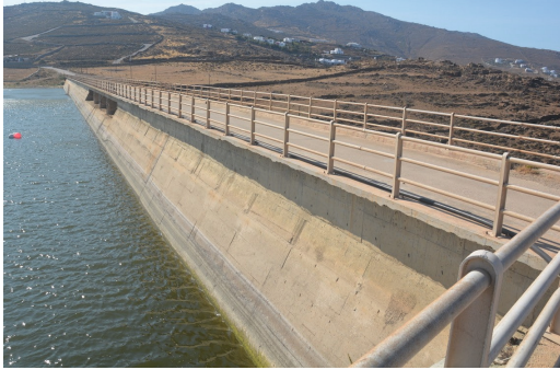
Marathia (Greece) – 1993: 1 st dam hard embankment; H = 31 m © M. Dunstan
