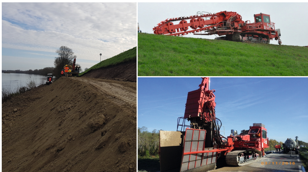
Figure 9.6 – Reinforcement works on the Loire side slope (left) and waterproof “deep soil mixing” screen in the levee of Orléans (right) / © DREAL Centre-Val de Loire
