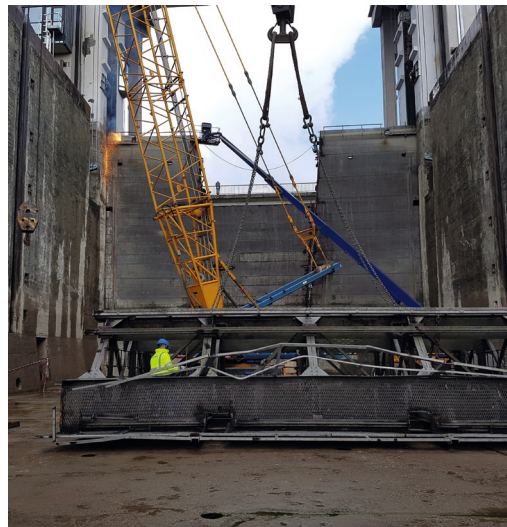
Figure 8.4 – Replacement of gates downstream of the lock chambers /
