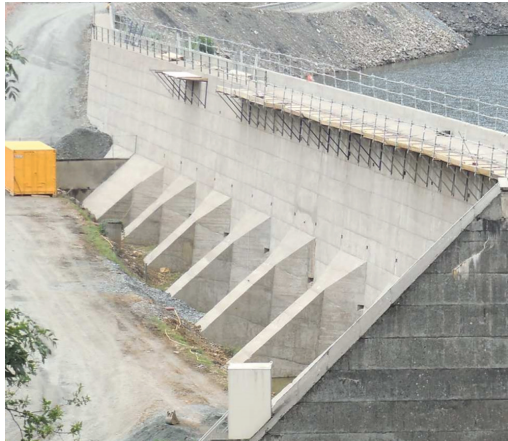
Figure 5.11 – Rassisse dam, stabilization by concrete backfill (left: before; right: after) / © ISL – Anthony Dols
