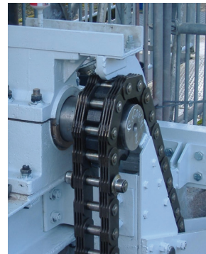
Figure 12.5 – Review of the condition of a Galle chain actuating a flood gate / © EDF
