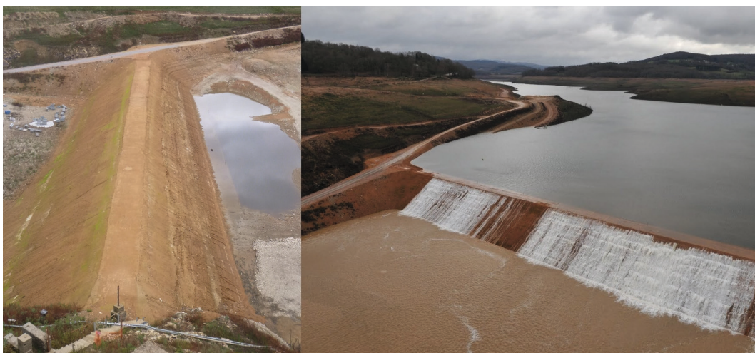
Figure 9.10 – Pannecière cofferdam being built et being overflowed / © BETCGB/ISL
