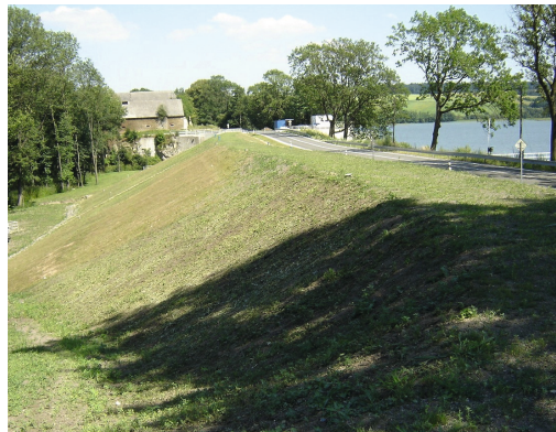
Figure 7.13 – Hvezda dike (Czech Republic, 2003) – General look of the dike after reconstruction / @ Lhoist
