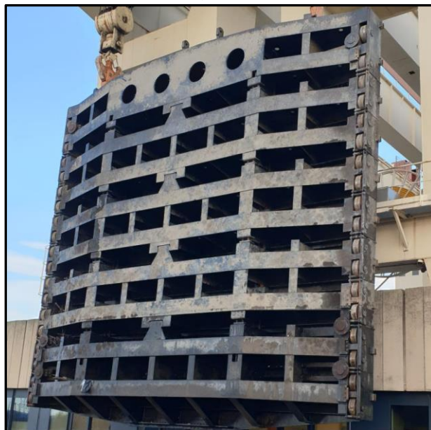
Figure 2: Vanne aval extraites de ces rainures
