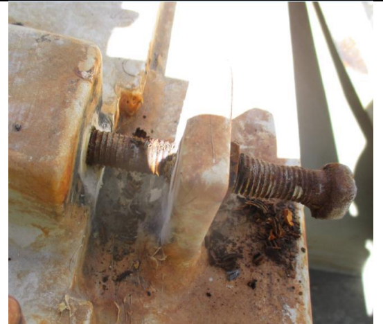
Figure 4 : vis de plaquage
