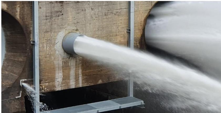
Figure 24 - Vanne jet creux en service (photos EIFFAGE)
