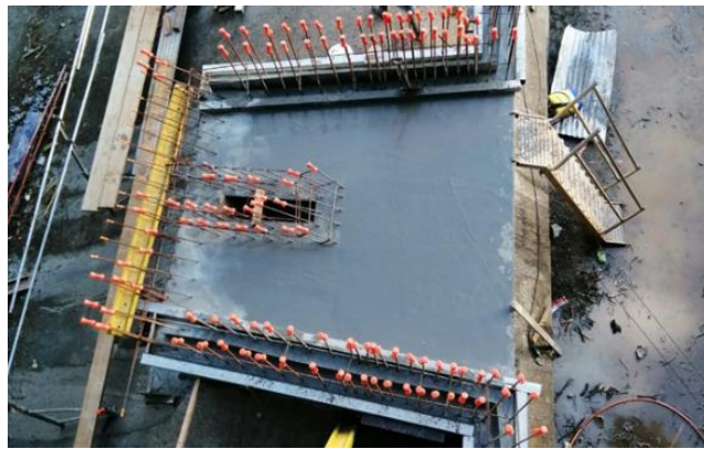
Figure 6. Installation de la base des Fusegate®
