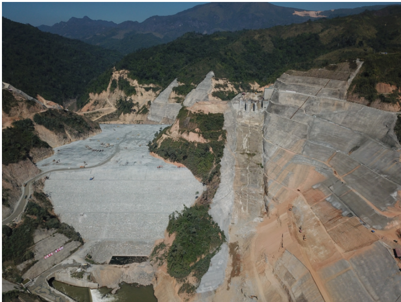
Downstream view of the dam and spillway
