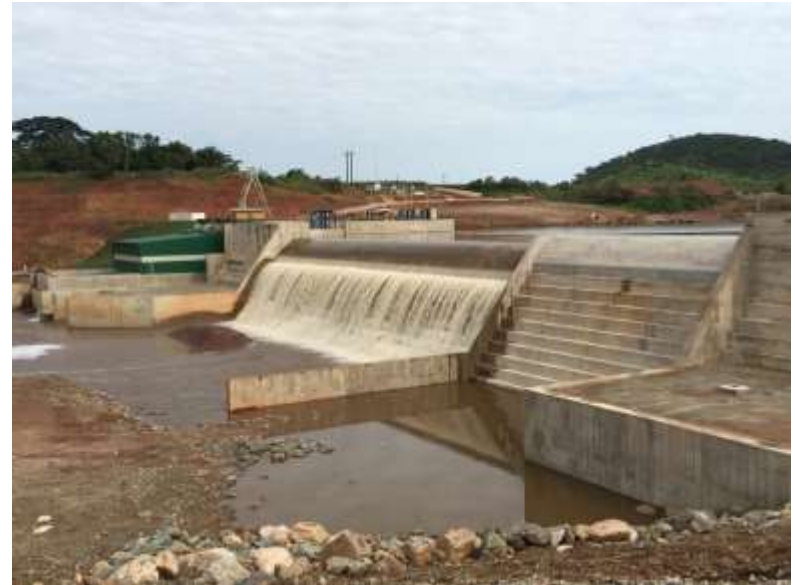
Amburau dam in RCD - 2016
